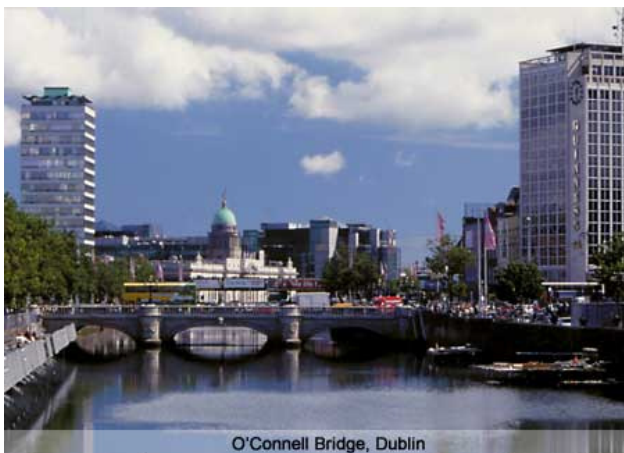
O'Connell Bridge, Dublin
